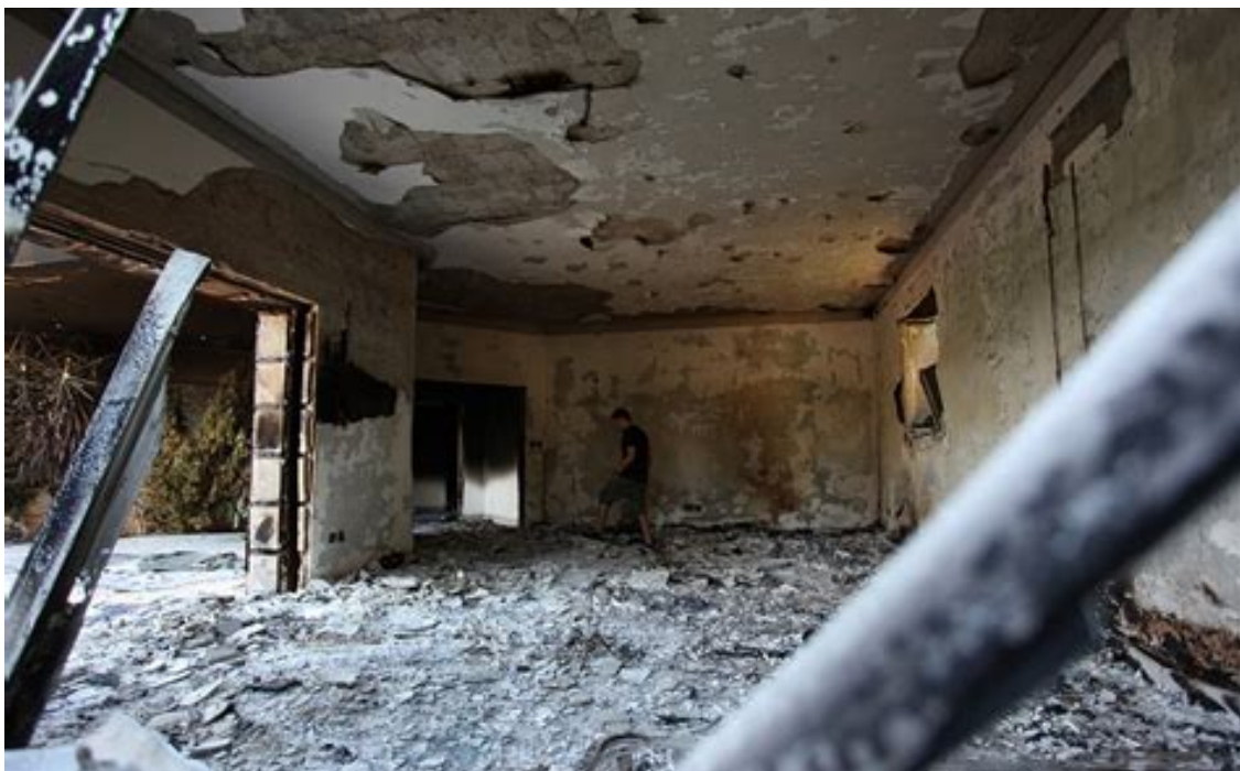
Remnants of Our Benghazi Consulate
